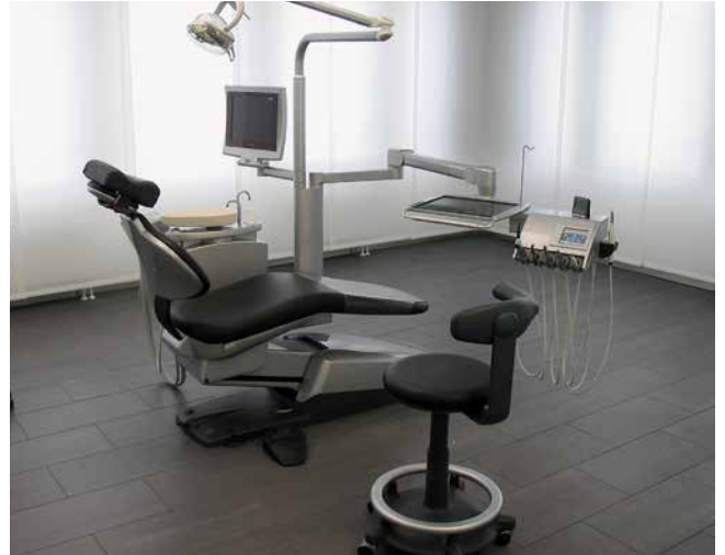
Medical facilities (treatment rooms etc.)
