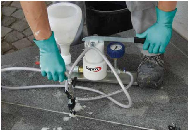
Void grouting with injection press (up to 15 bar)
