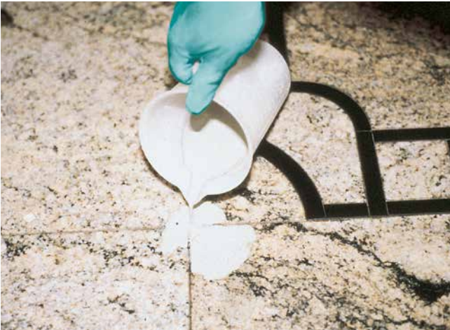
Filling of voids via open joint.
