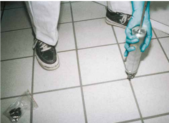
Small-scale void grouting using hand syringe.
