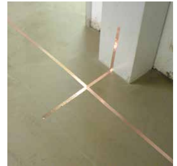
Copper strip laid on floor surface.
