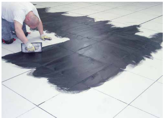
6 Floor covering grouted using Sopro FL plus with Sopro ELD 458 conductive dispersion as additive.
