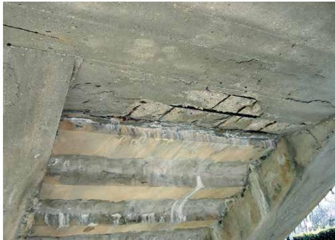
Corrosion damage to a stair soffit caused by lack of waterproofing and inadequate concrete cover.
