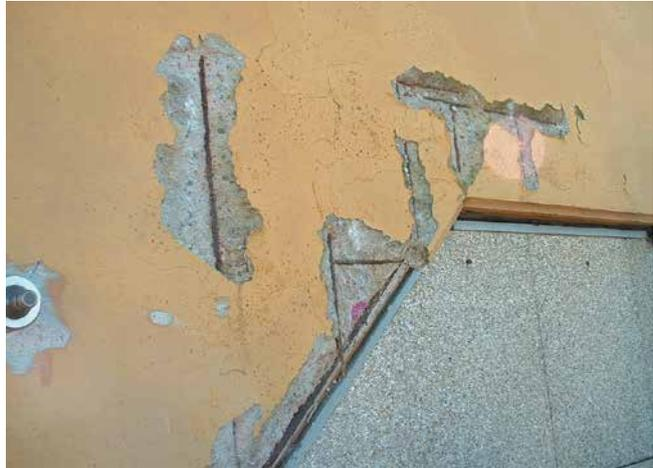
Spalling on a facade due to inadequate concrete cover.
