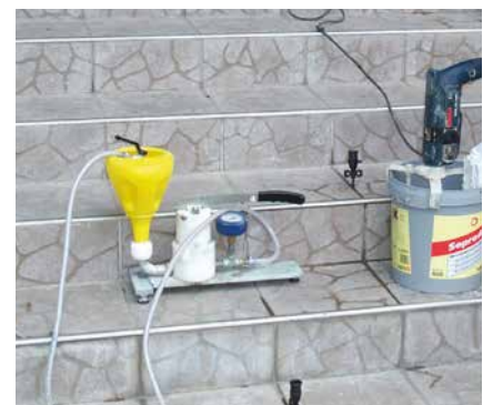
Grouting of voids below stair covering.
