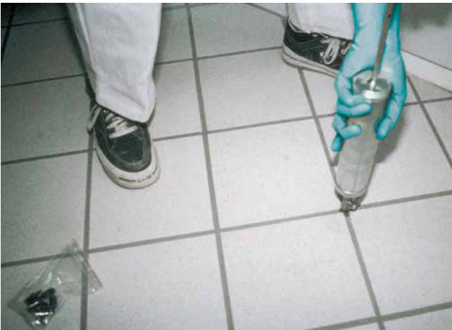
Small-scale void grouting using hand syringe.
