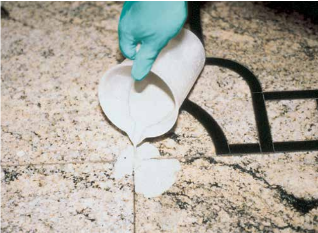
Filling of voids via open joint.
