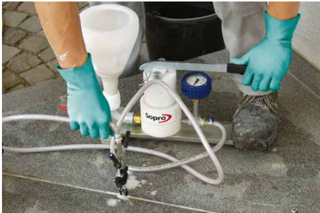
Void grouting with injection press (up to 15 bar).
