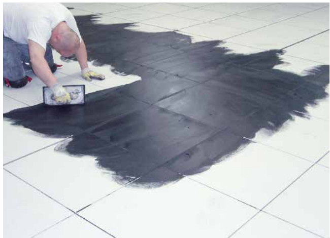
6 Floor covering grouted using Sopro FL plus with Sopro ELD 458 conductive dispersion as additive.
