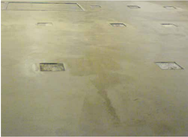
1 Floor levelled using Sopro FS 15 550 and primed to receive covering.
