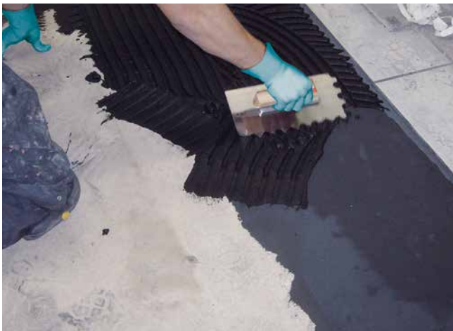
5 Ceramic covering laid using thin-bed adhesive with electrically conductive additive.
