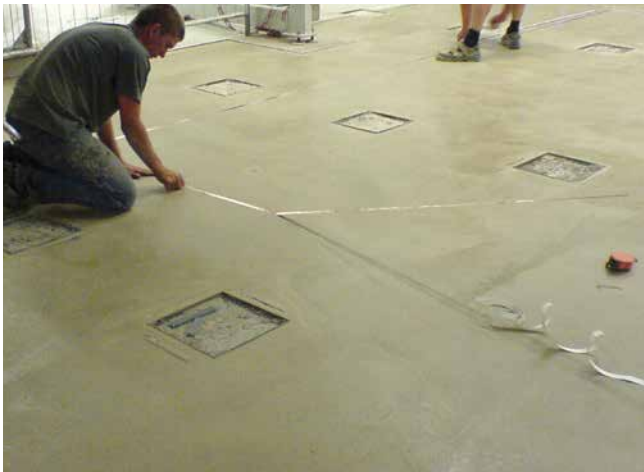
3 Copper strip fixed in accordance with required grid size.
