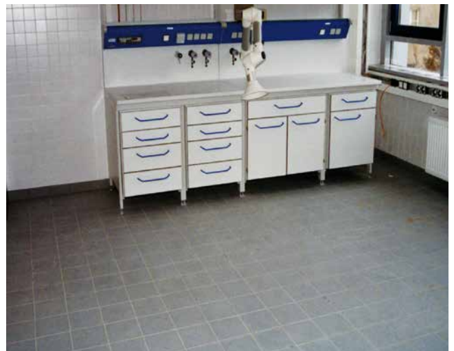
Laboratory space subject to explosion hazards
