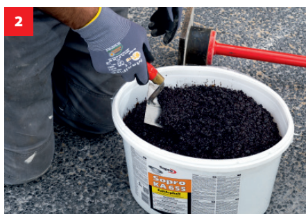
2 V fuge nanosite Sopro hladno asfaltno zmes,
